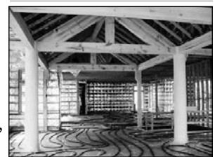
Typical slab layout using 7/8" Pex tubing.
