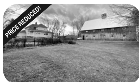
Derby Gorgeous barn, salt water pool, landscaped 1.06A Main St. lot. The 3-BR/3-BA home, in need of restoring, has many salvageable items. NOW $265,000 Nick - #4849635
