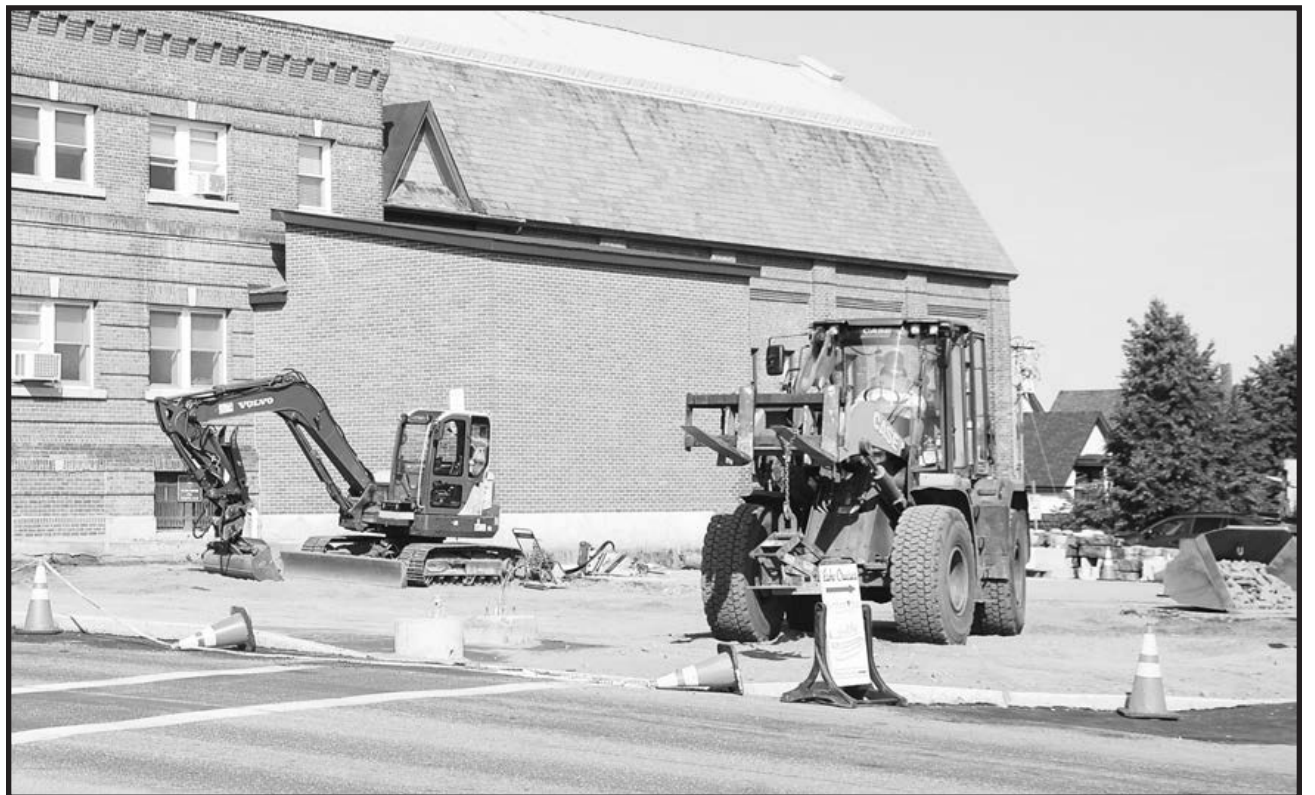
Machines prep the municipal building's former parking area for construction.
